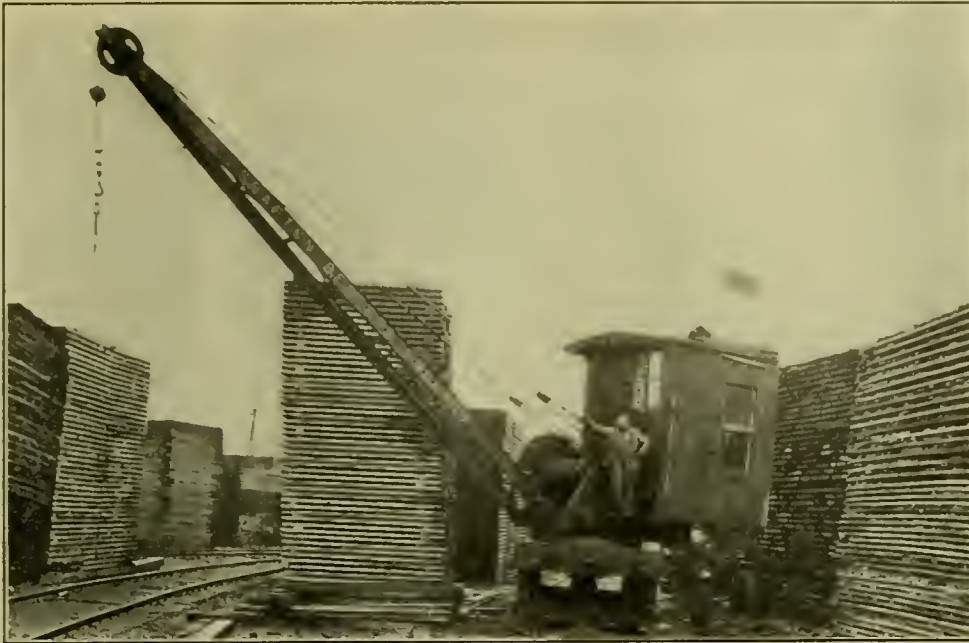
FIG. 45.—FIVE TON GRAFTON CRANE IN THE LUMBER YARD.
